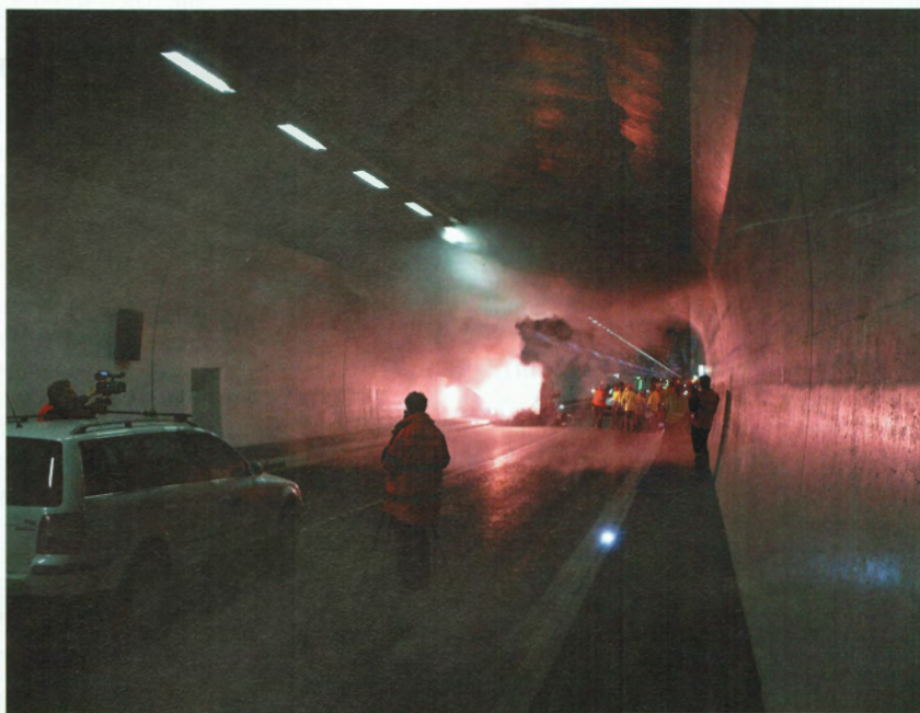
Above: Smoke testing exercises underway in tunnels.
