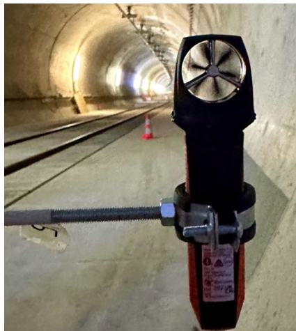
Figure 9: Vane anemometer fixed to a grid frame in a rail tunnel
