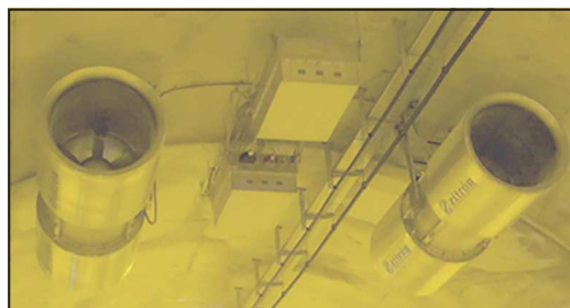
Figure 13. Jet fans and control units in the Polana tunnel
