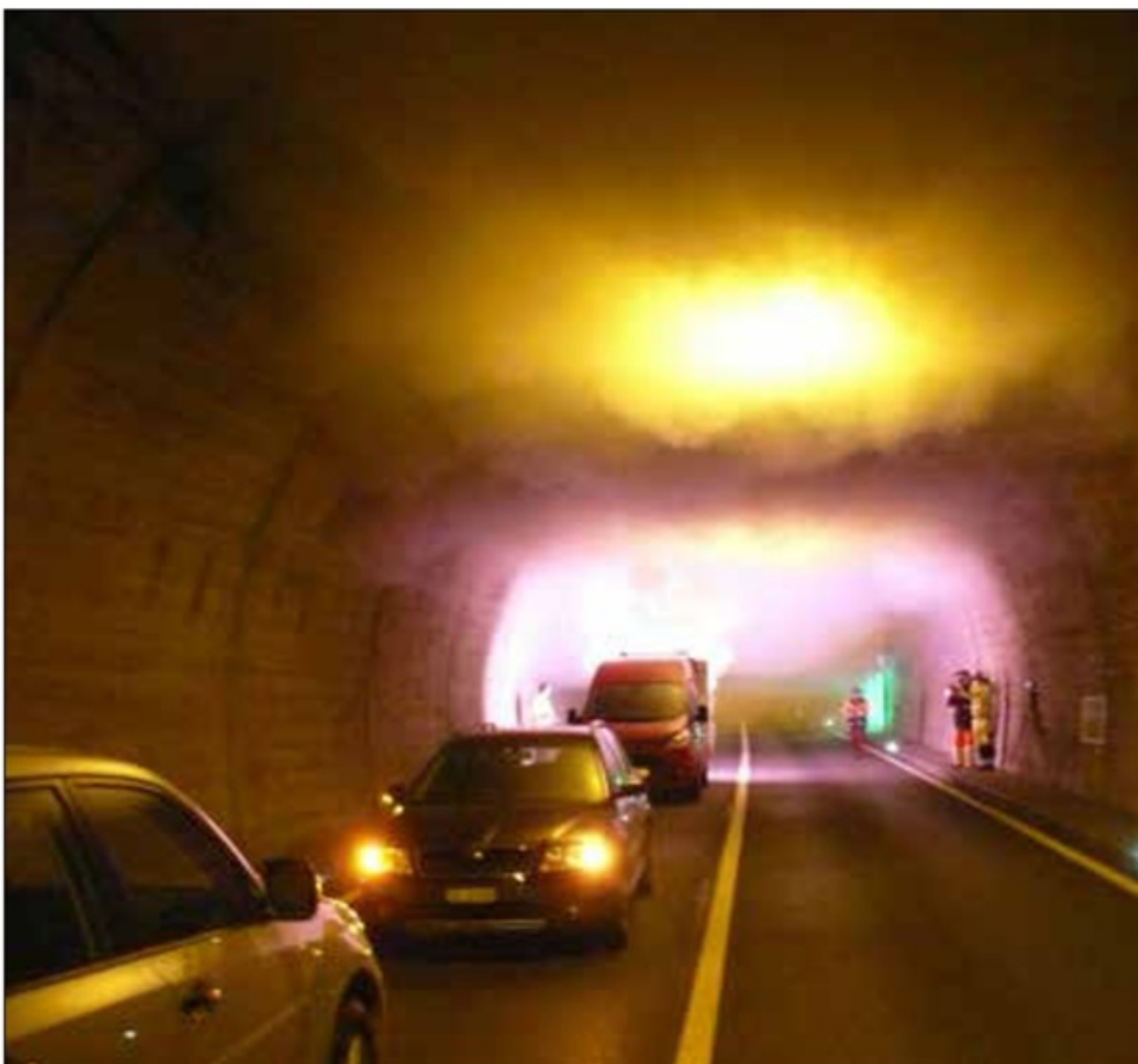
Figure 5: Controlled smoke layering during a hot smoke test in a road tunnel
