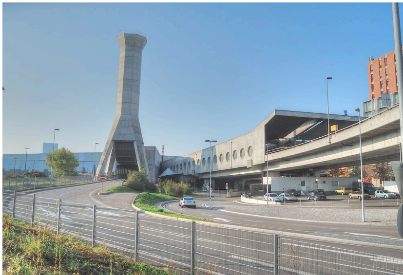
Figure 5: Obsolete Ventilation Shaft of Nordtangente Tunnel, Basel, Switzerland
