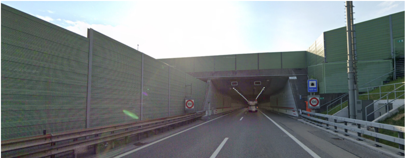
Figure 2 Tunnel portal with absorptive noise protection panels
