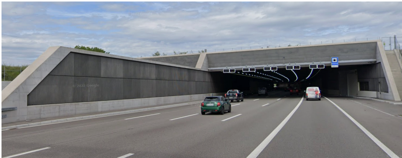
Figure 1 Highway lid, built under traffic (Zurich North Bypass, Switzerland)
