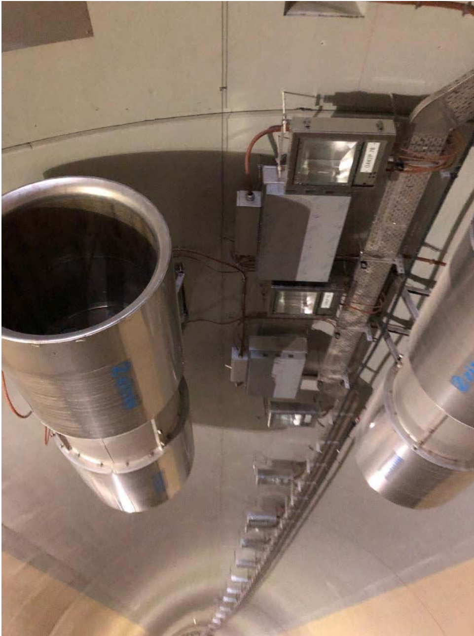
Figure 5. Jet fans with in-tunnel control units
